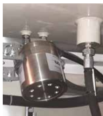
Fire extinguishers mounted and aligned by means of pivoting console clamps
