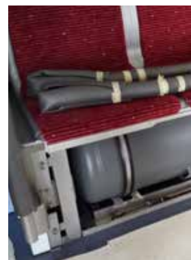
Under-floor installation of supply lines with HY-ROS system mounts
